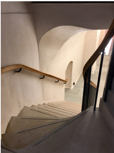
The new SW Staircase
